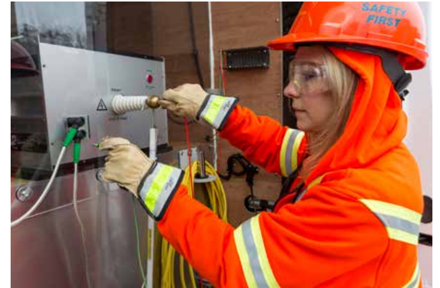
Alana Jones, a test engineer for Energy Ottawa, performs a cable test.
